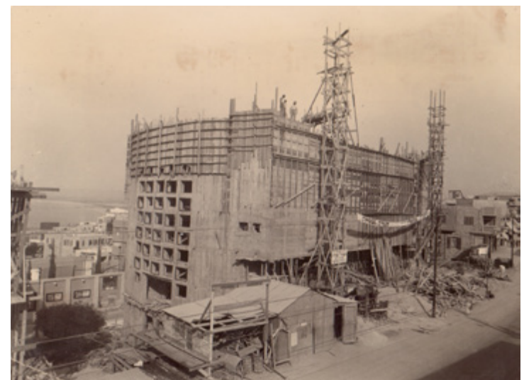
The Ora Cinema under construction, 1935. Photo: Fernbach and Fuchs, courtesy Solei Boneh
