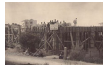
Construction of Bet Hapoalim, the Nachman Syrkin Workers' House, 1926. Courtesy Solel Boneh Archive
